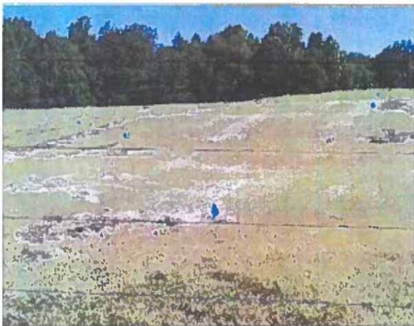
Adequate site prep requires the removal of existing vegetation, like this turf grass, without which, wildflower seedlings would have to compete with the existing vegetation for sunlight, water, and nutrients. (Photograph courtesy of Don Keirstead, New Hampshire NRCS)
